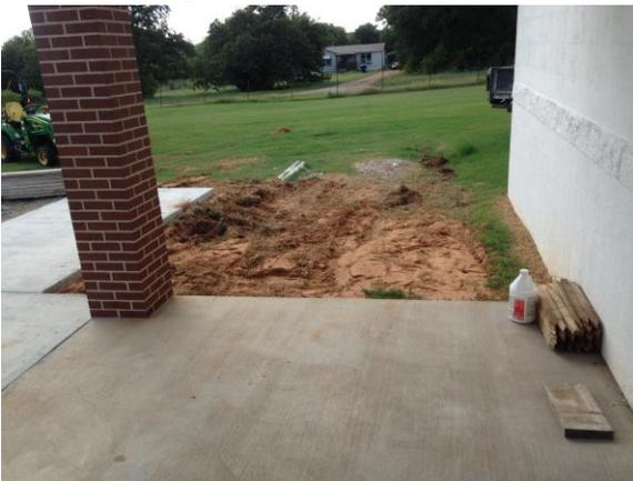
our last big rains washed all the dirt from under the new sidewalk so we dug and poured a stem wall around the side walk. This seems to be working. It will look a lot better after we get all the dirt filled in.
